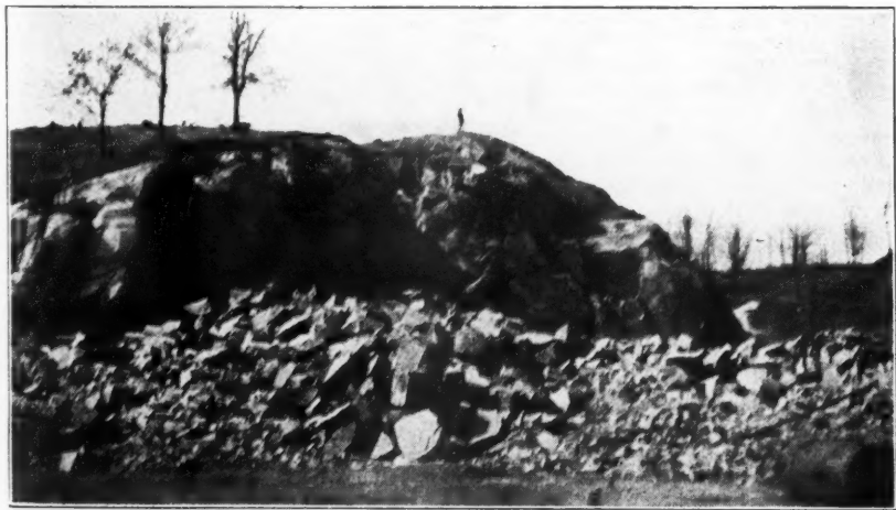
Lower Face of Quarry Worked Only for Paving Blocks
